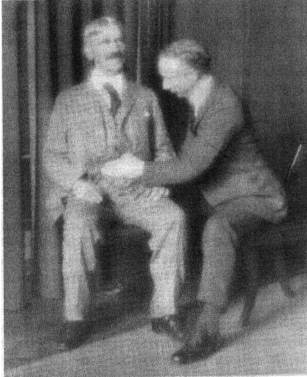
Another photo taken by Irene Tasker of Alexander working with John Dewey from 1916/1917. Here Alexander works with Dewey from a seated position. Note Dewey's outward gaze. Is Alexander "widening the back" from the floating ribs?
